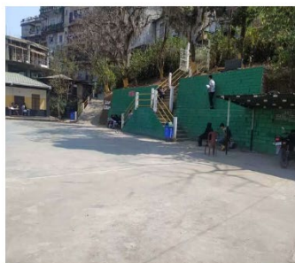
Pu R Vanlalvena MLA pawhin Concrete Retaining wall a siam sak
